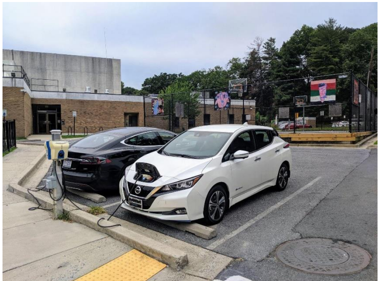
Figure 1, EVI AC Level 2 charging stations in-use (Source: PlugShare)
